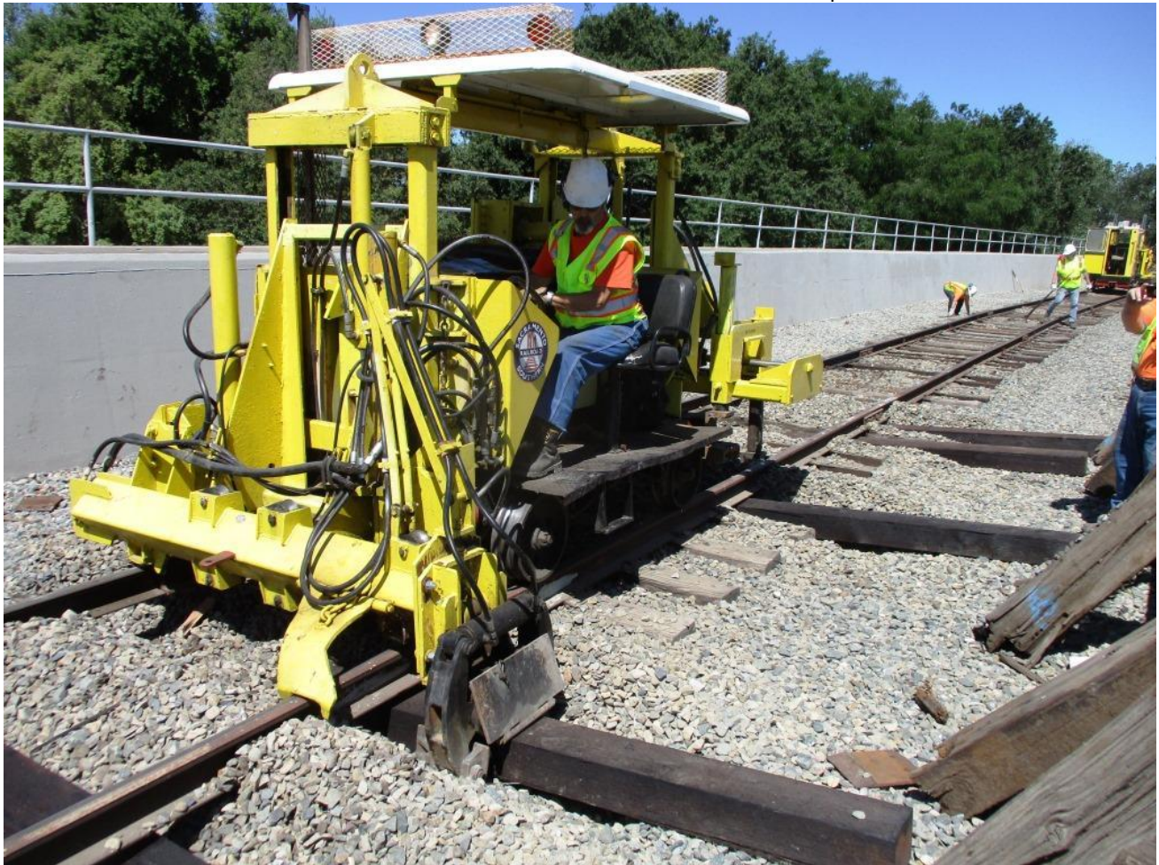
Ed on the 125 now pulls the new ties into place
