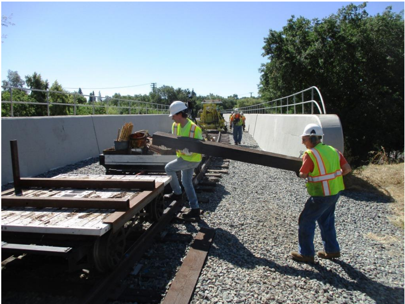
Hemi and Clem move a tie from the truck to the flatcar
