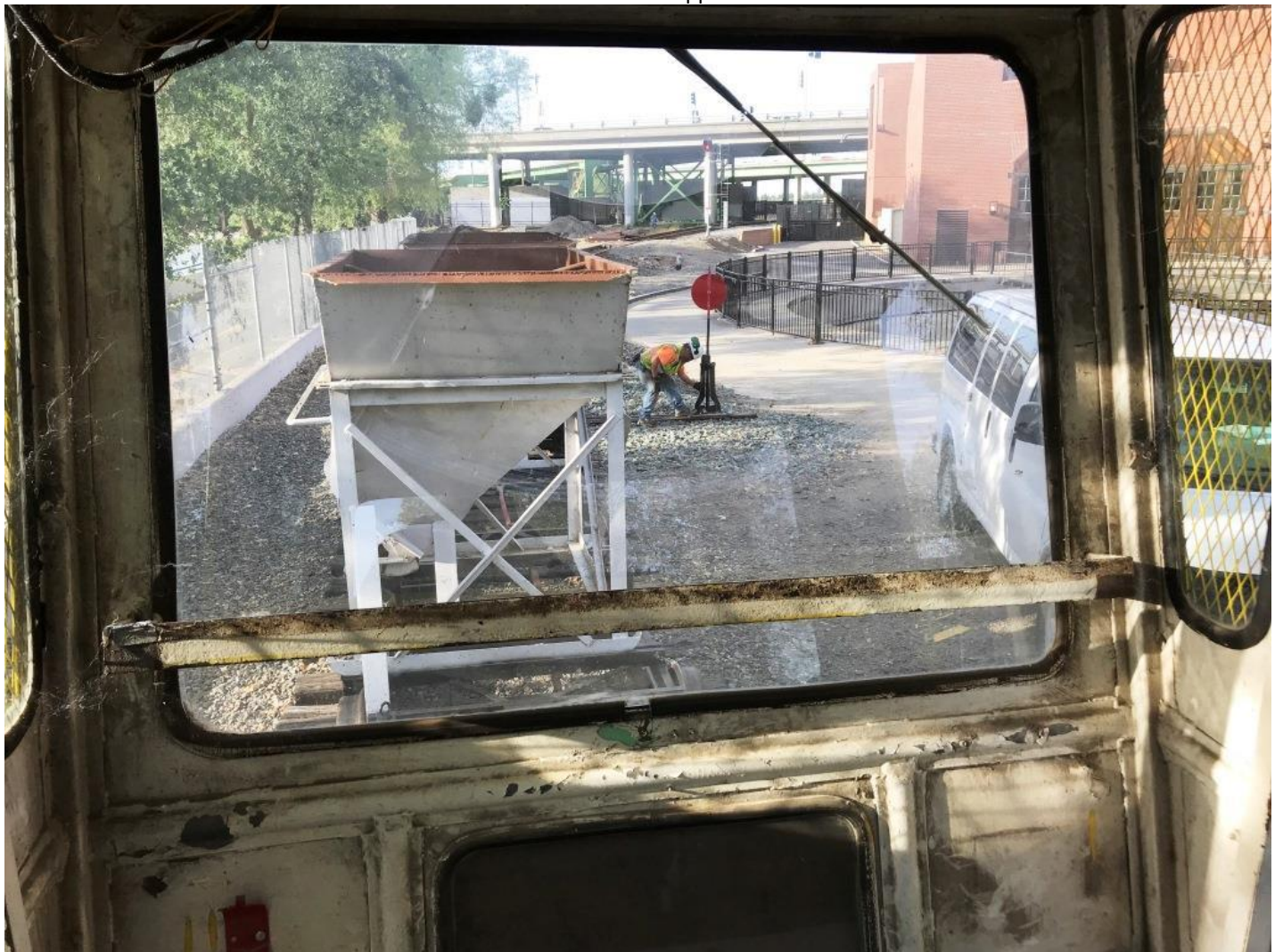
Joe switches the ballast regulator and hoppers onto the 560 Track
