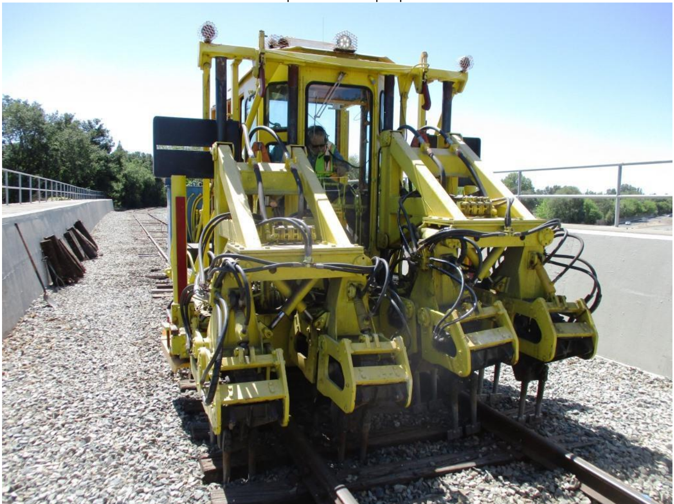
Alan tamps the bridge track
