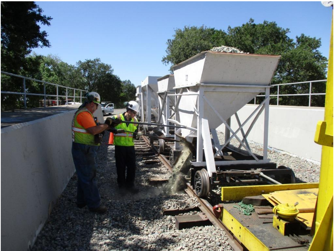
Mike F. and Jack discharge rock from the other side-dump car
