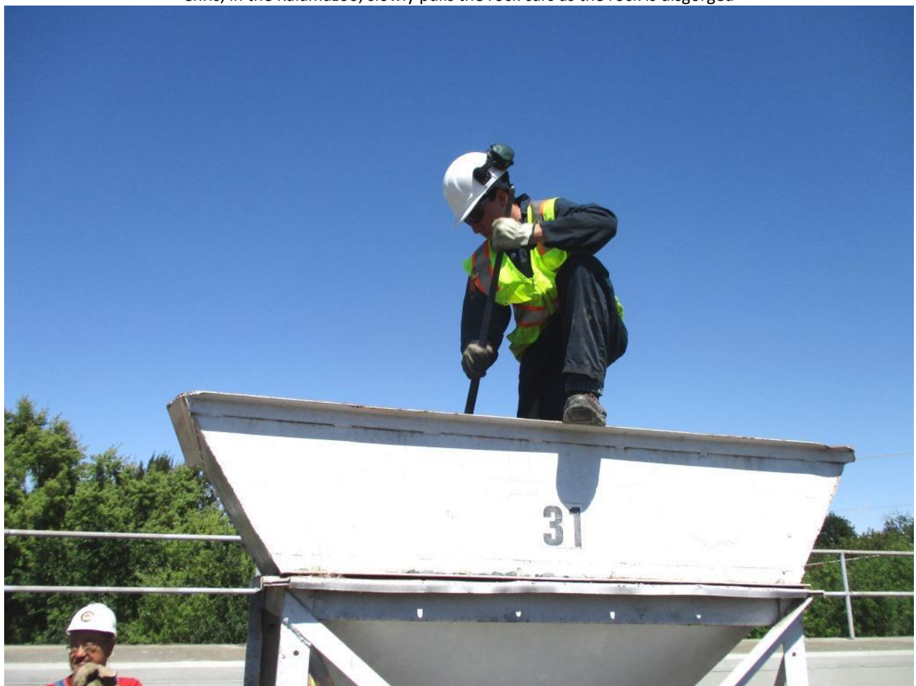
Jack climbs up into the hopper and uses a lining bar to unplug the jammed-up rock
