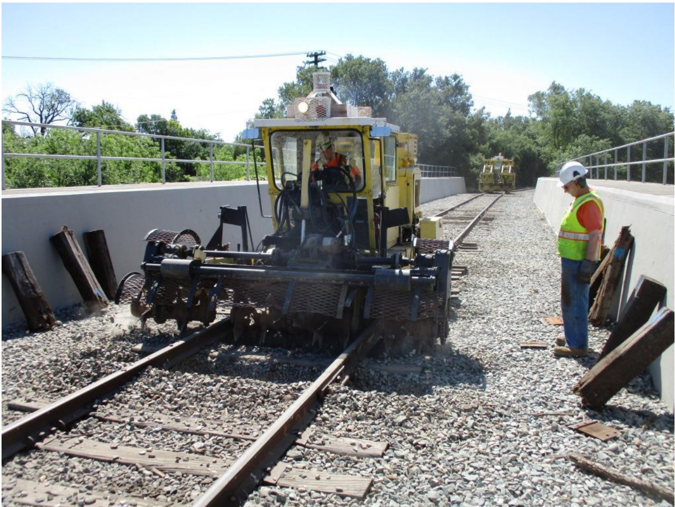
After Frank had chopped the ties up with the tie-shear, Clem guides Mike F. in the scarifier as he digs new tie-cribs
