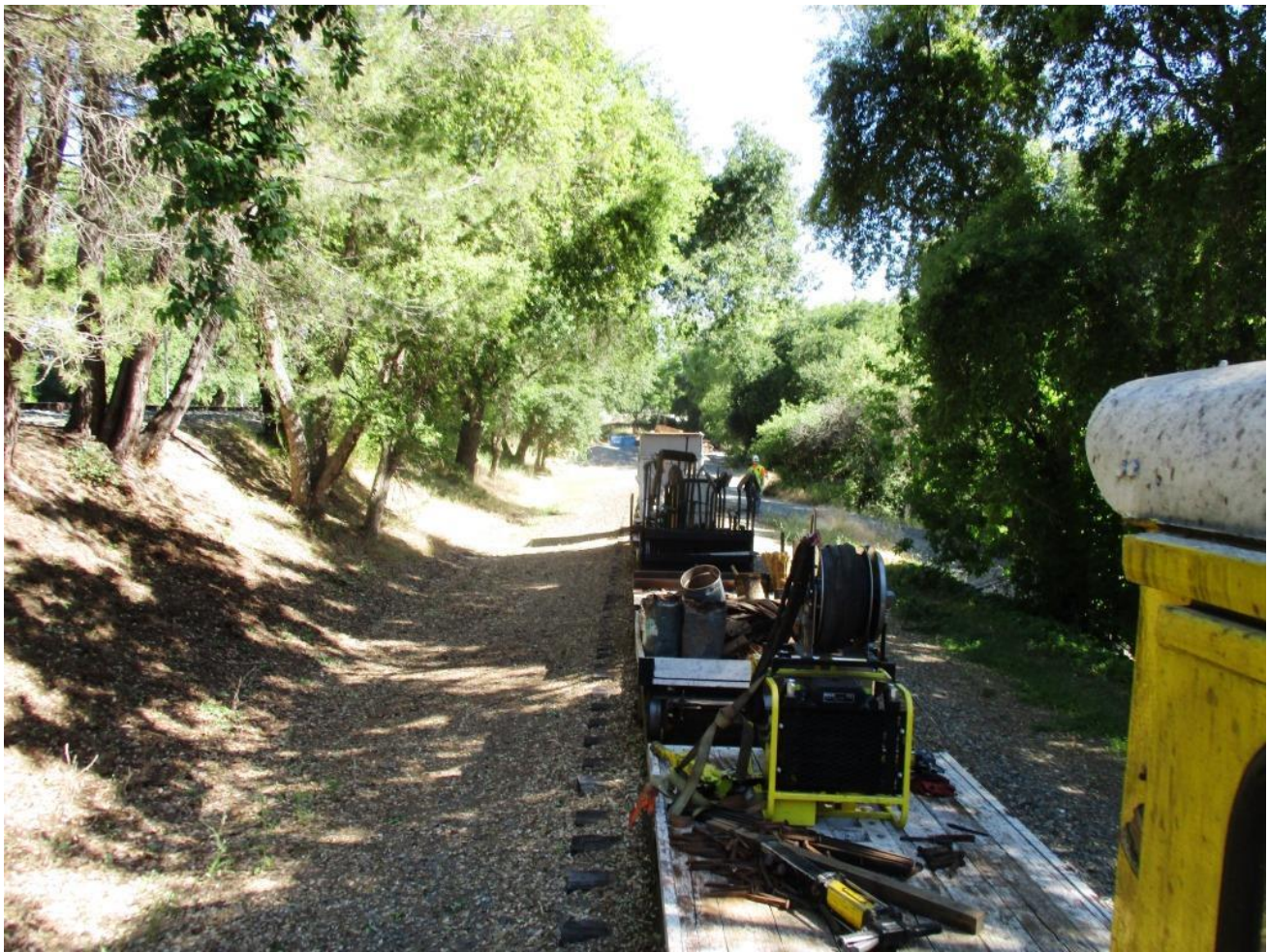
Chris walks the point of the work-train as the second set of hoppers are deposited at Setzer for Harry on the back-hoe to fill
