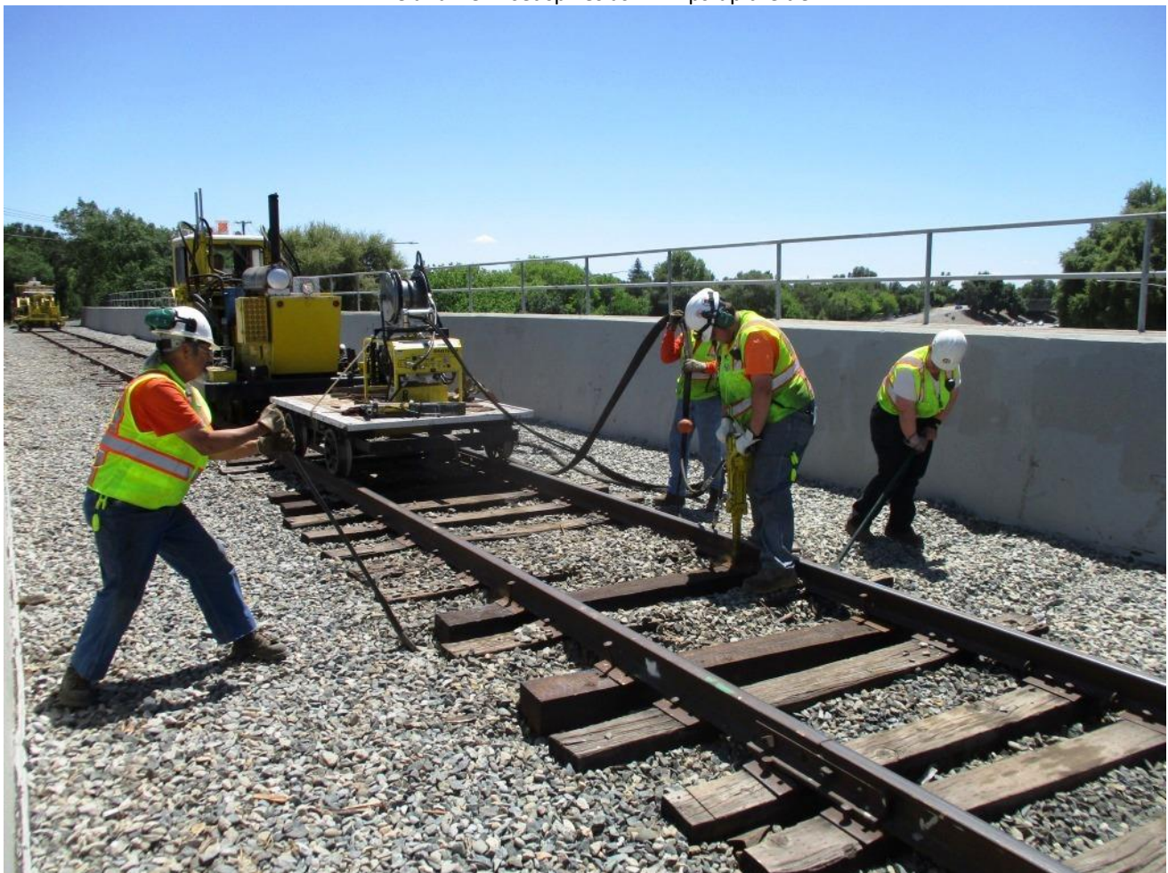
Ed and Heather nip the tie as Chris drives spikes with the hydraulic spike driver
