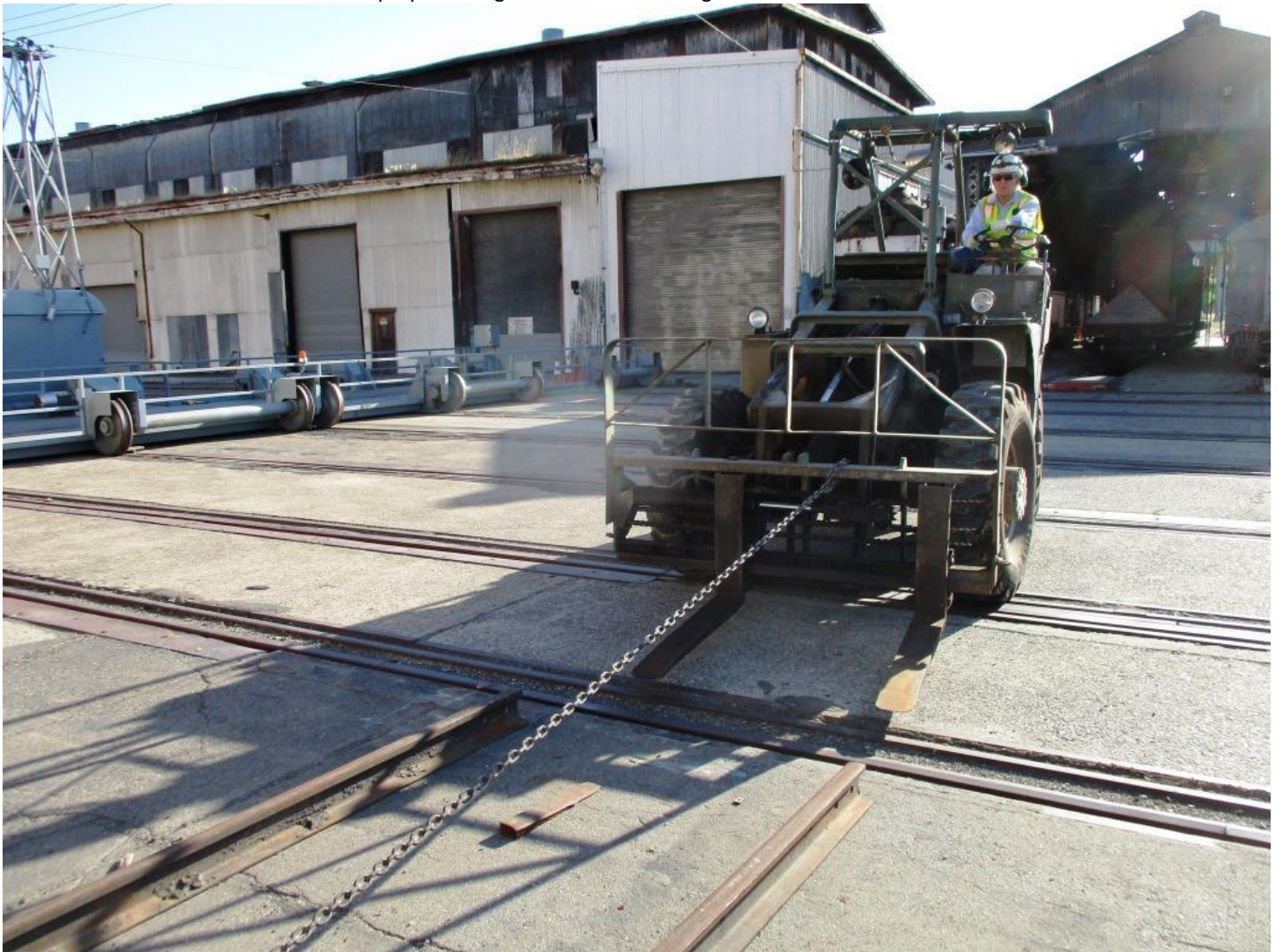
Steve, on the Big Green Machine, attempts to pull the snap track closer to the transfer table runway to close the gap
