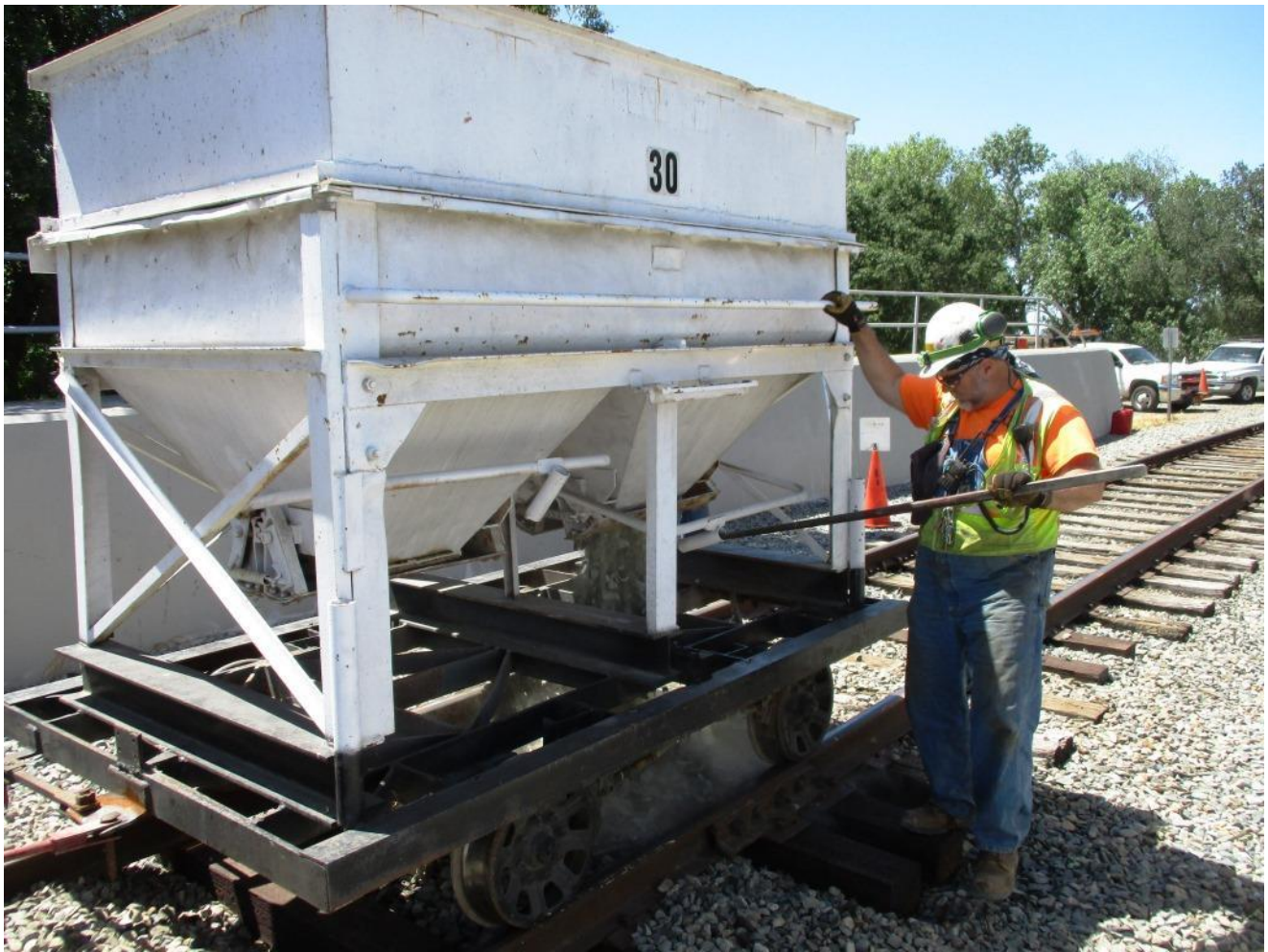
Mike F. starts the ballasting process by disgorging rock from the center-dump hopper car
