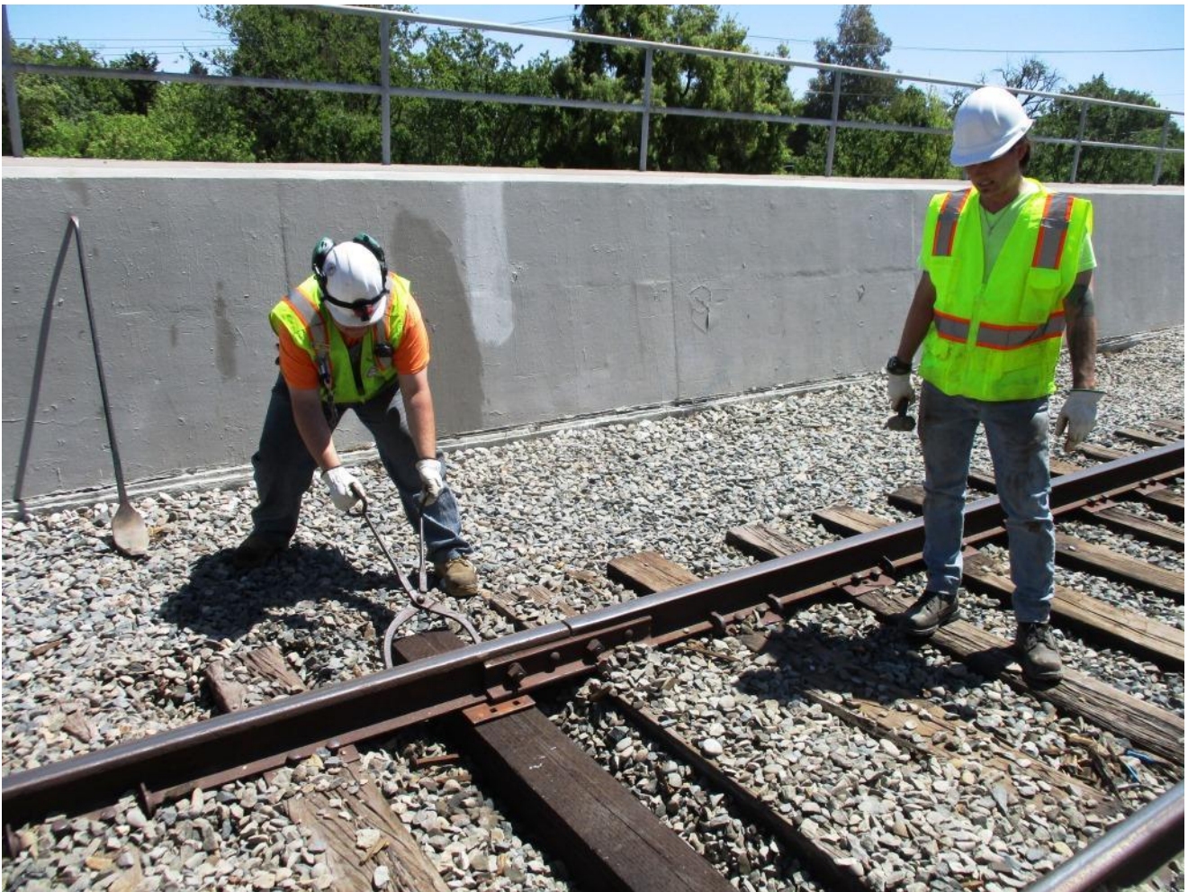
Chris repositions the tie to make sure it is centered
