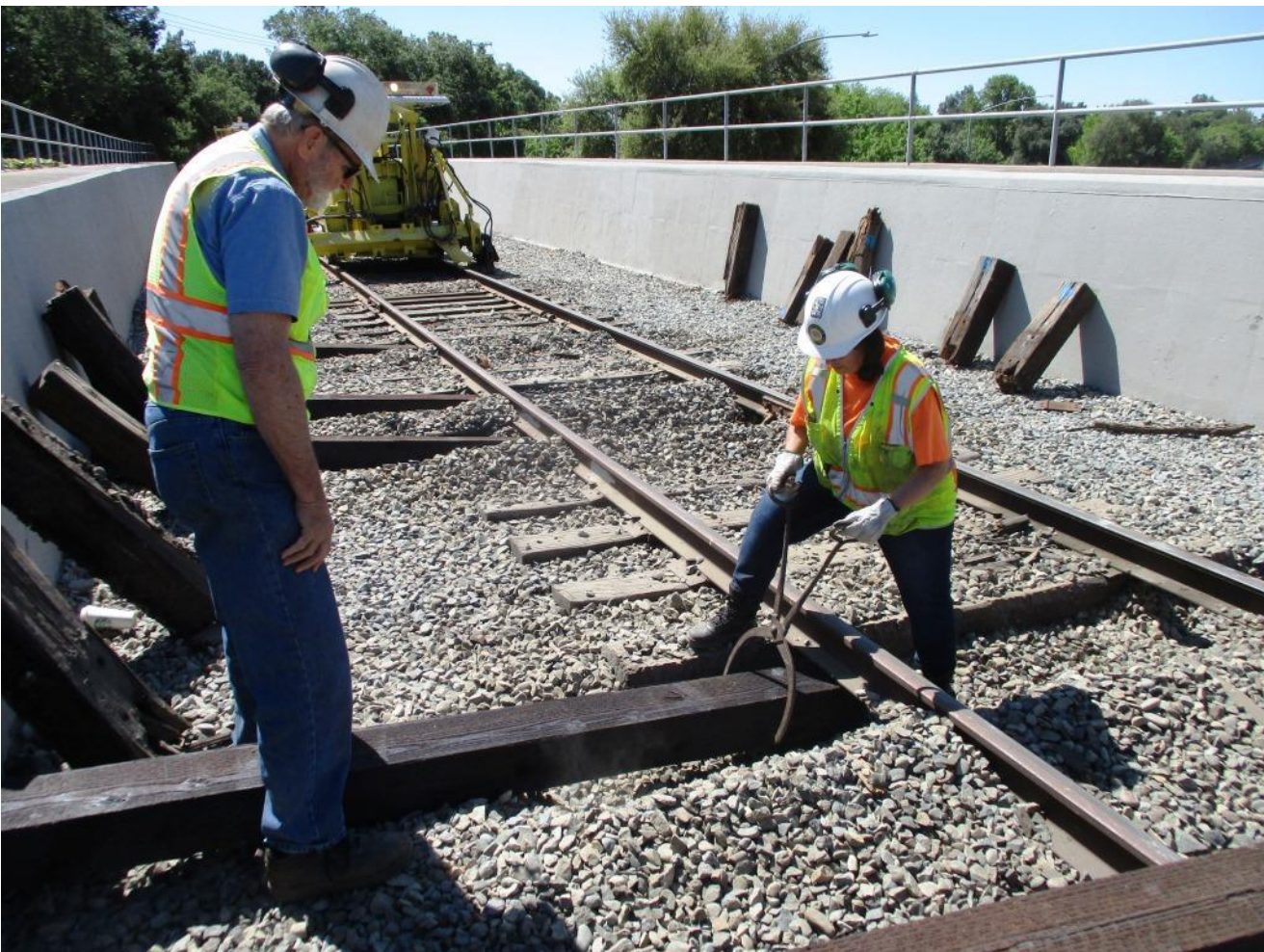
Pam uses tie-tongs to position the end of the tie under the base of the rail
