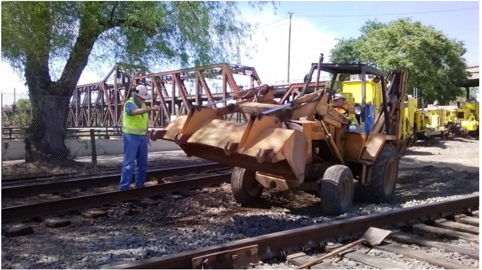
Alan and Mike H. prepare the ground for the building of a new switch behind the Museum
