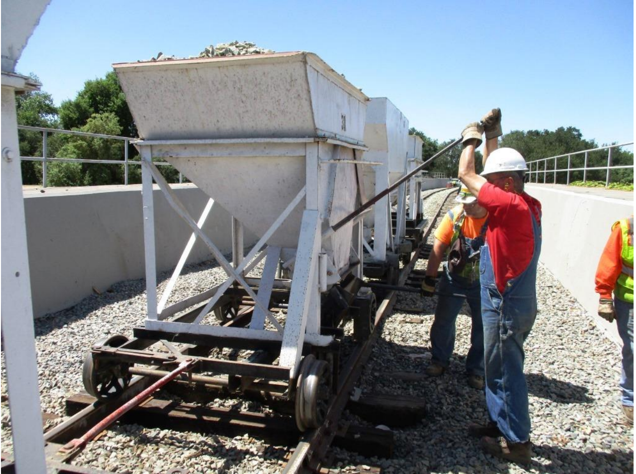
John and Mike H. disgorge rock from the side-dump car
